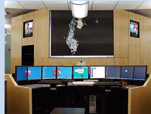
Secure Critical Infrastructure
